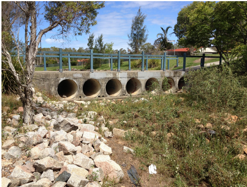
Photograph looking upstream at structure
