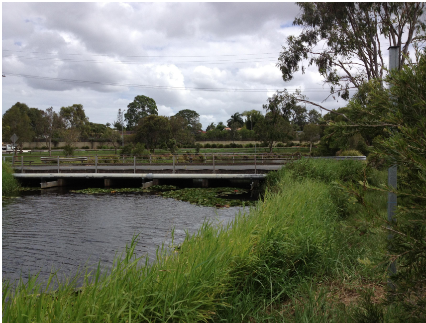
Photograph looking upstream at structure
