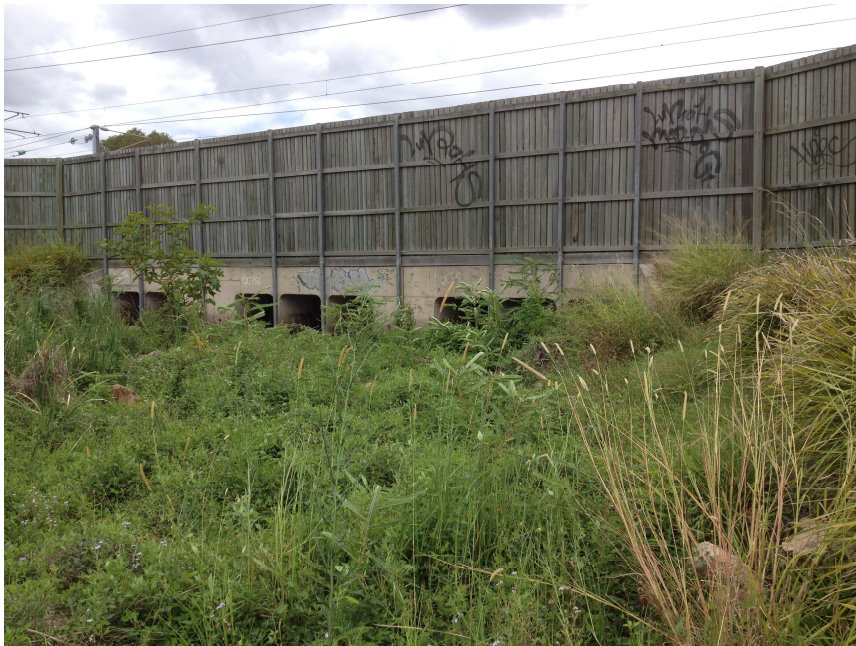
Photograph looking upstream at structure
