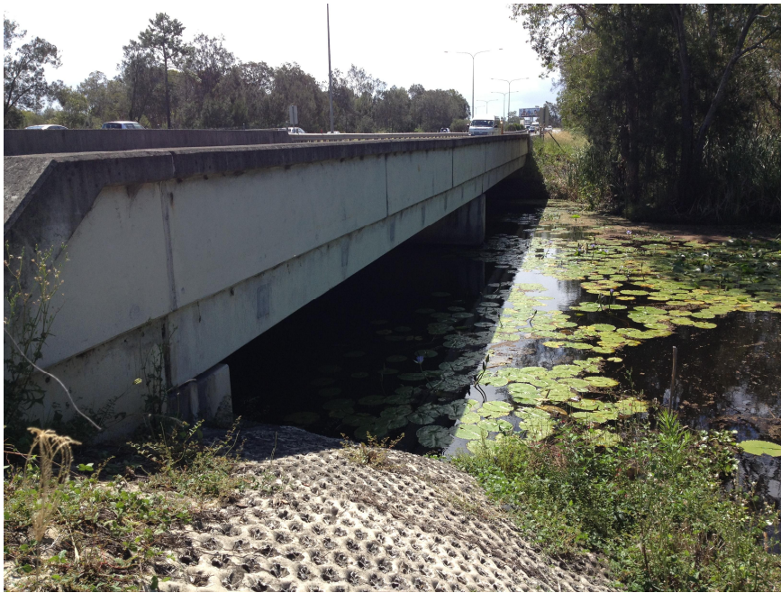
Photograph looking upstream at structure
