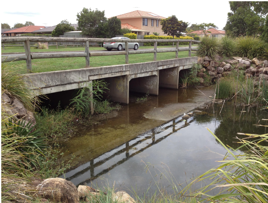
Photograph looking upstream at structure
