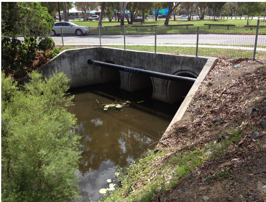
Photograph looking downstream at structure
