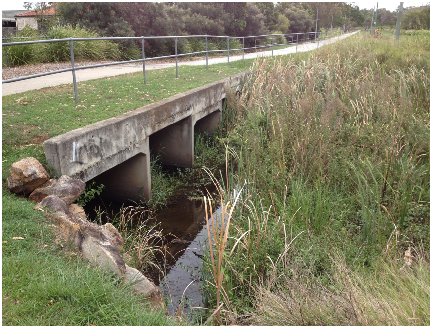
Photograph looking upstream at structure
