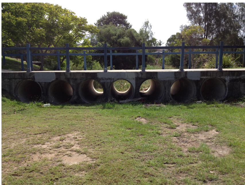
Photograph looking downstream at structure
