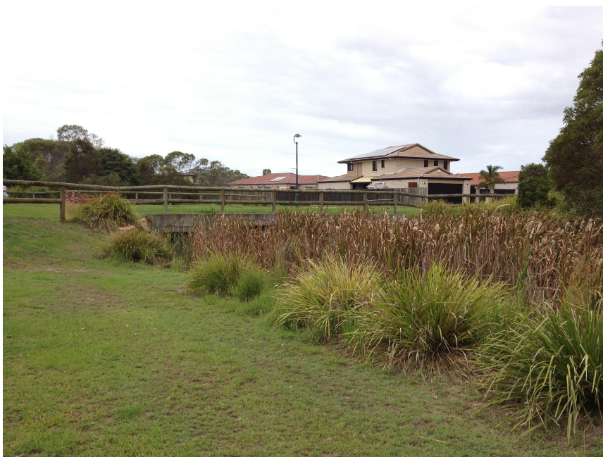
Photograph looking downstream at structure
