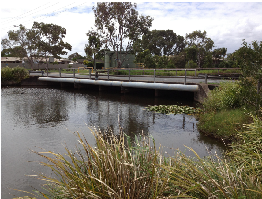
Photograph looking downstream at structure
