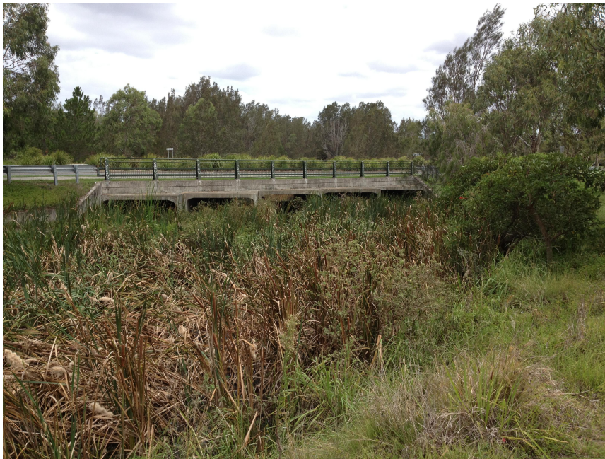
Photograph looking upstream at structure
