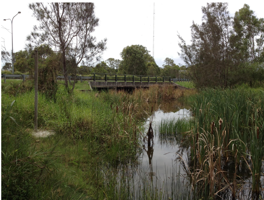
Photograph looking downstream at structure
